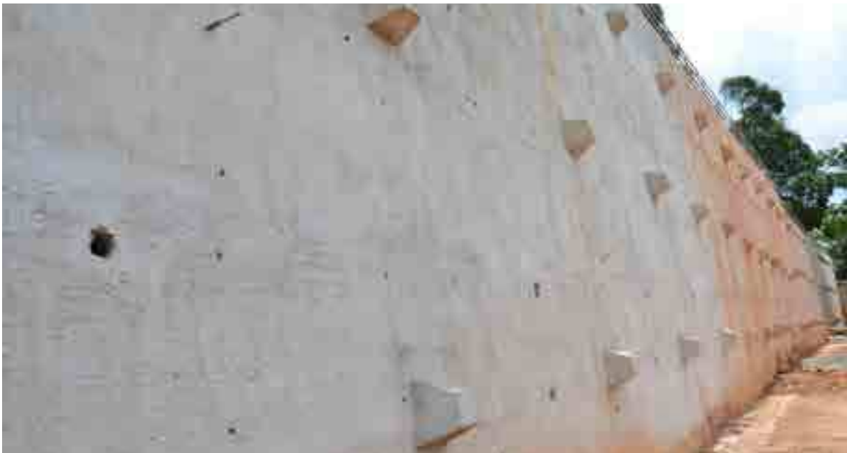
Muro de Contenç3o | Rua Vale Alegre Can3o
